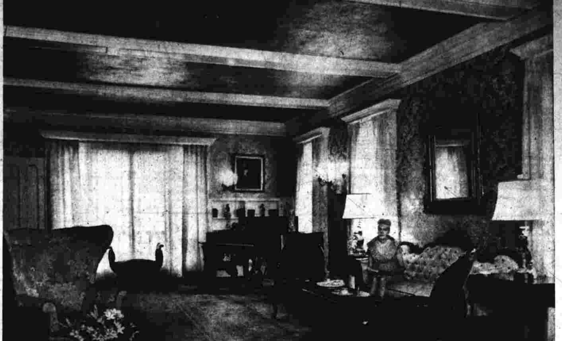
Residence of Mr. and Mrs. Frank H. Reed, 65 Prospect St.
